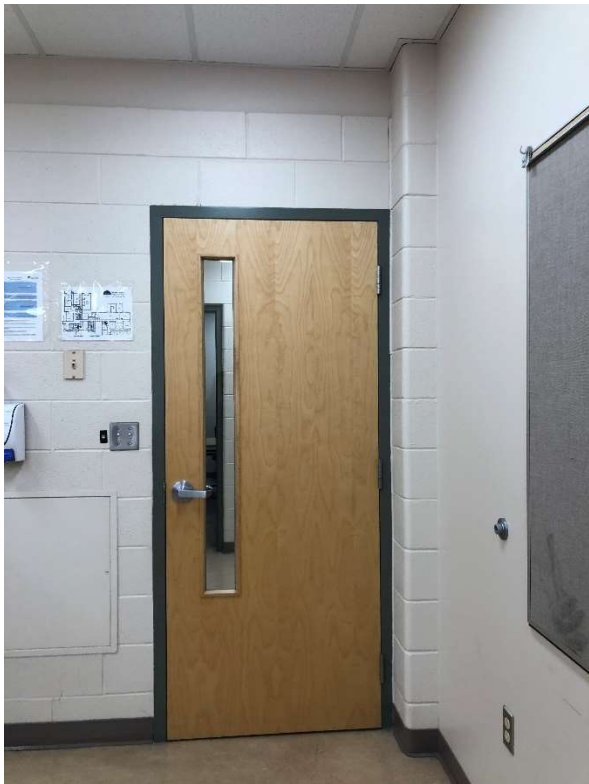
Photo 4: Existing Hall door to be removed
