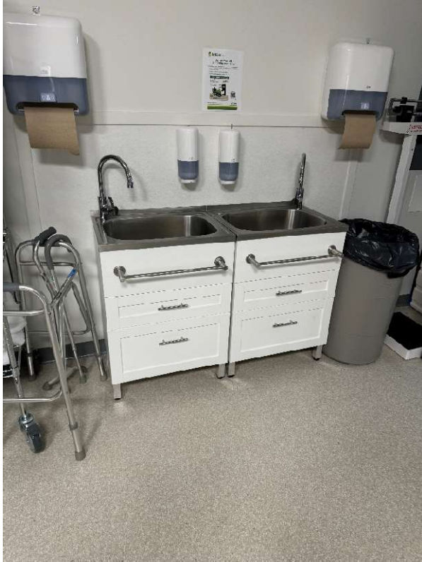
Photo 3: existing sinks to match
